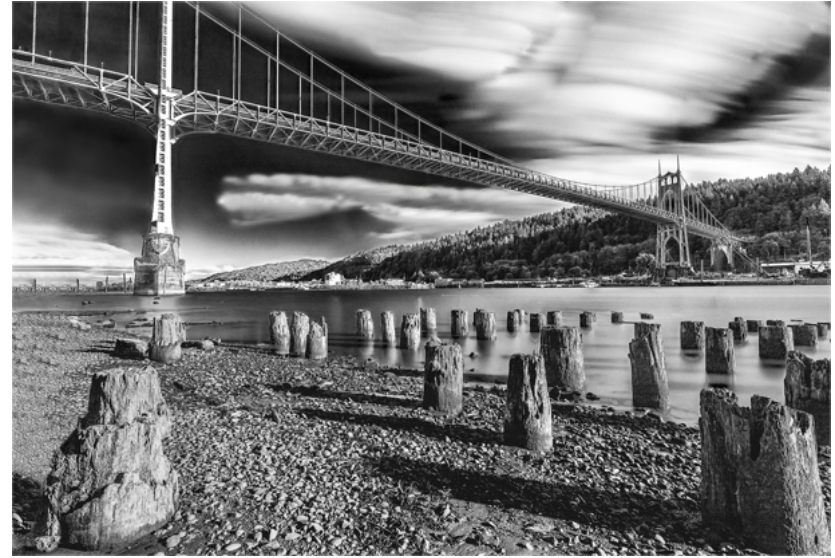
St. Johns Bridge by Doug Fischer
